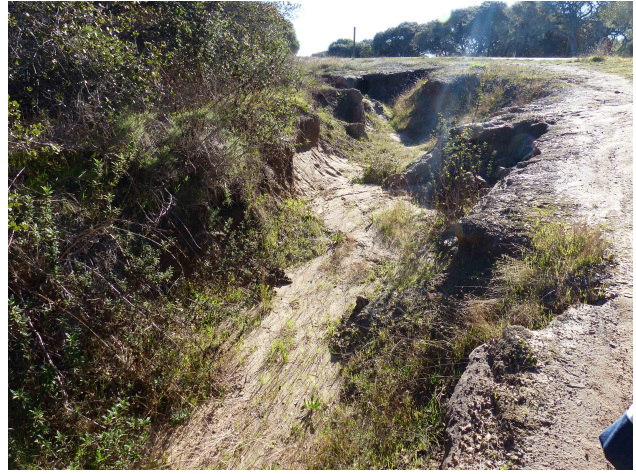
Erosion Feature - Gullying
